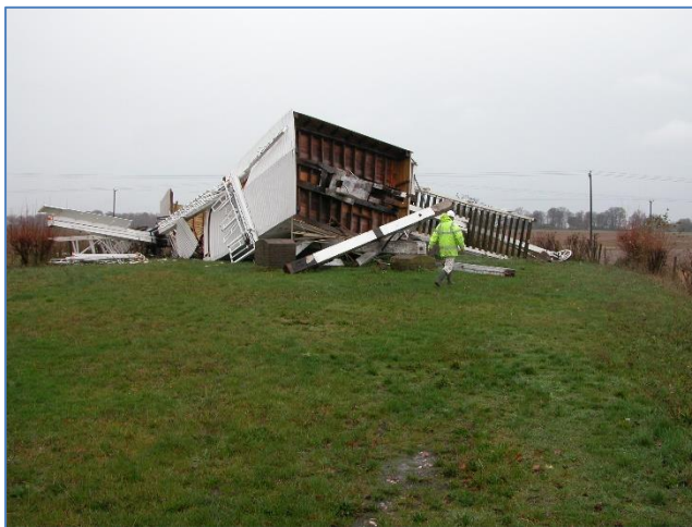
Figure 5 Chillenden windmill, blown down in 2003, now re-built
